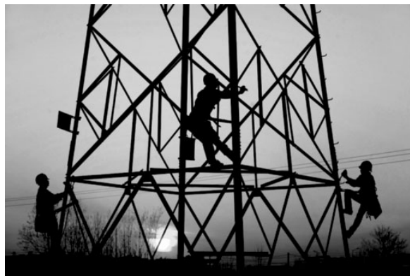
All the existing power sector reforms schemes, namely Deen Dayal Upadhya Gram Jyoti Yojana, Integrated Power Development Scheme and PM-KUSUM scheme, would be subsumed into this umbrella programme
